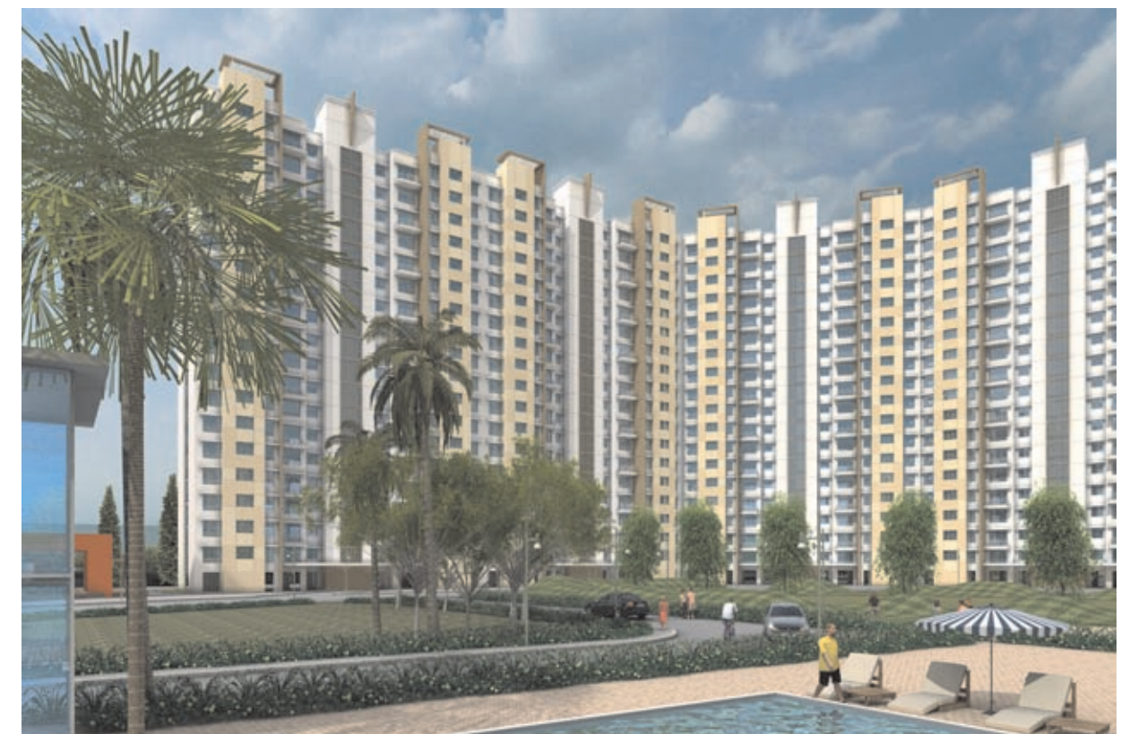
3 BHK TOWERS - CLUBHOUSE SIDE
